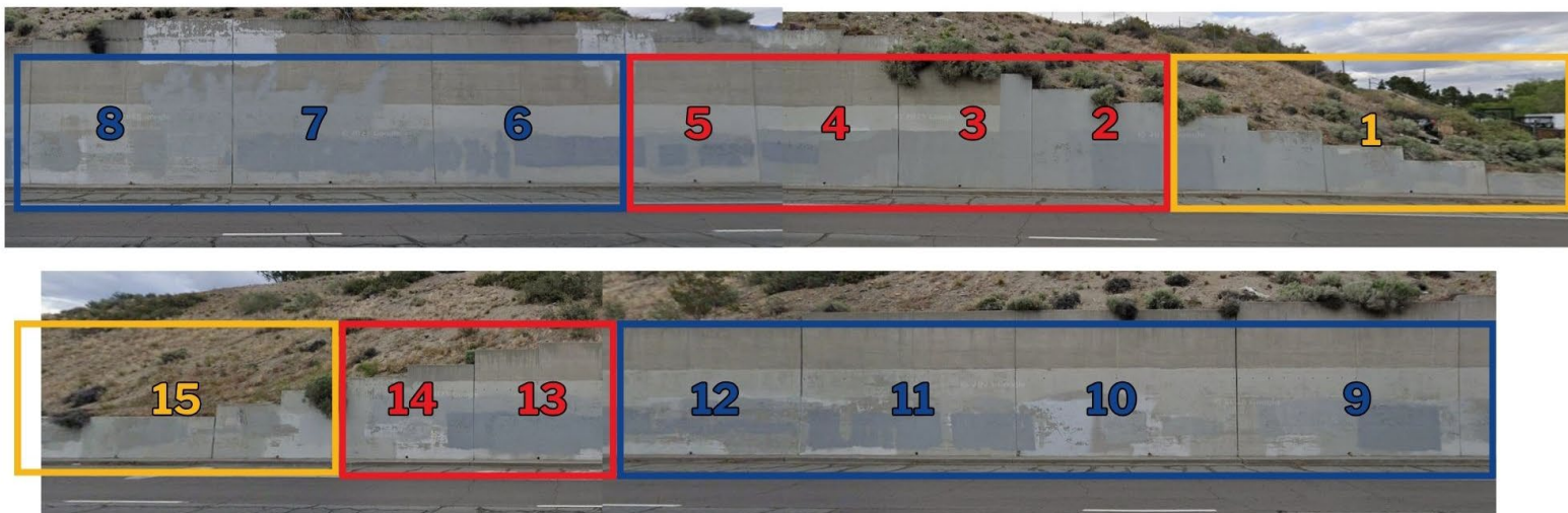
Pictured: West 4 th Street Retaining Wall Showing 15 Sections for 2026 Small Walls Program
